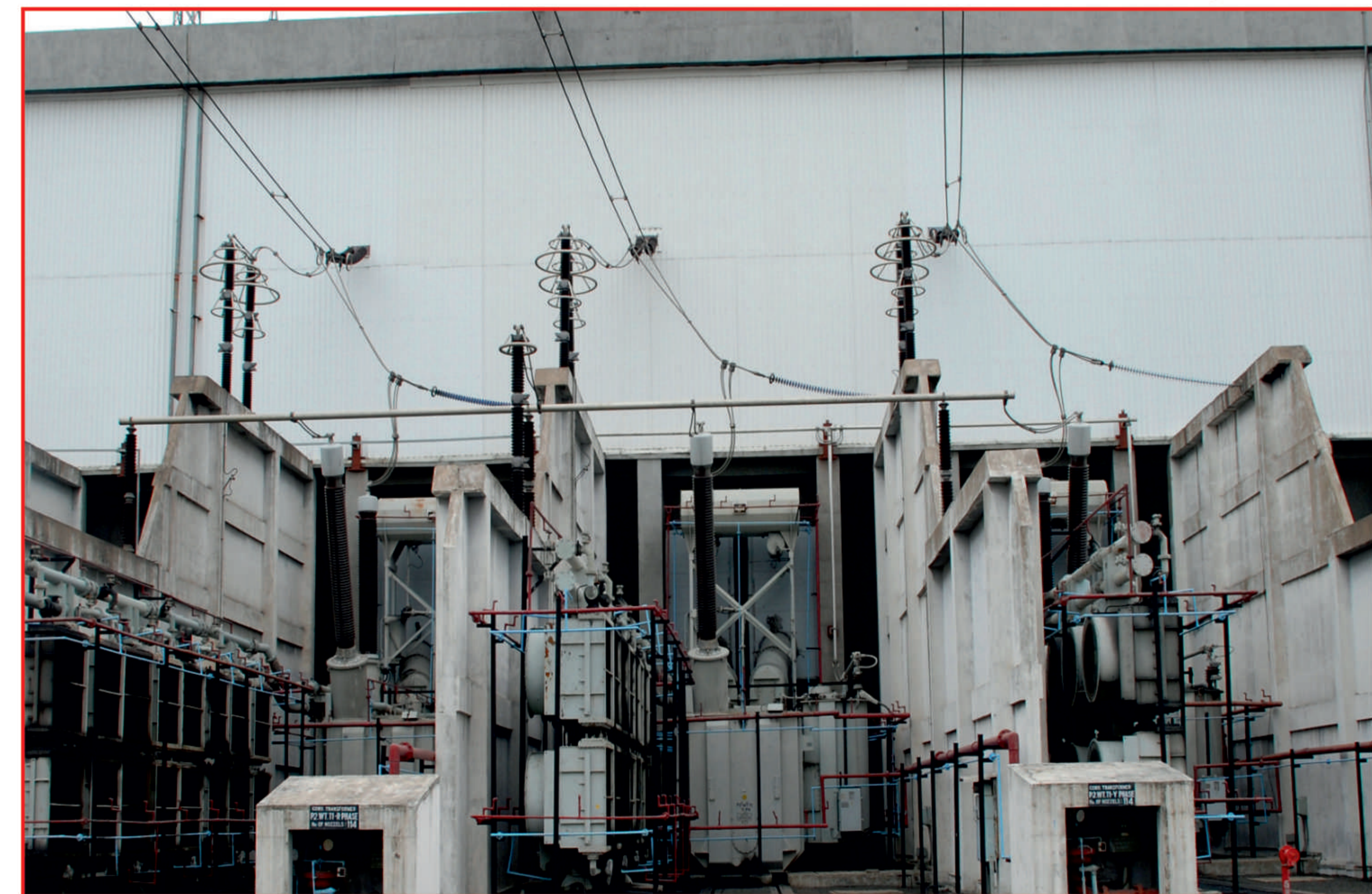
Converter Transformer at HVDC Station Chandrapur
