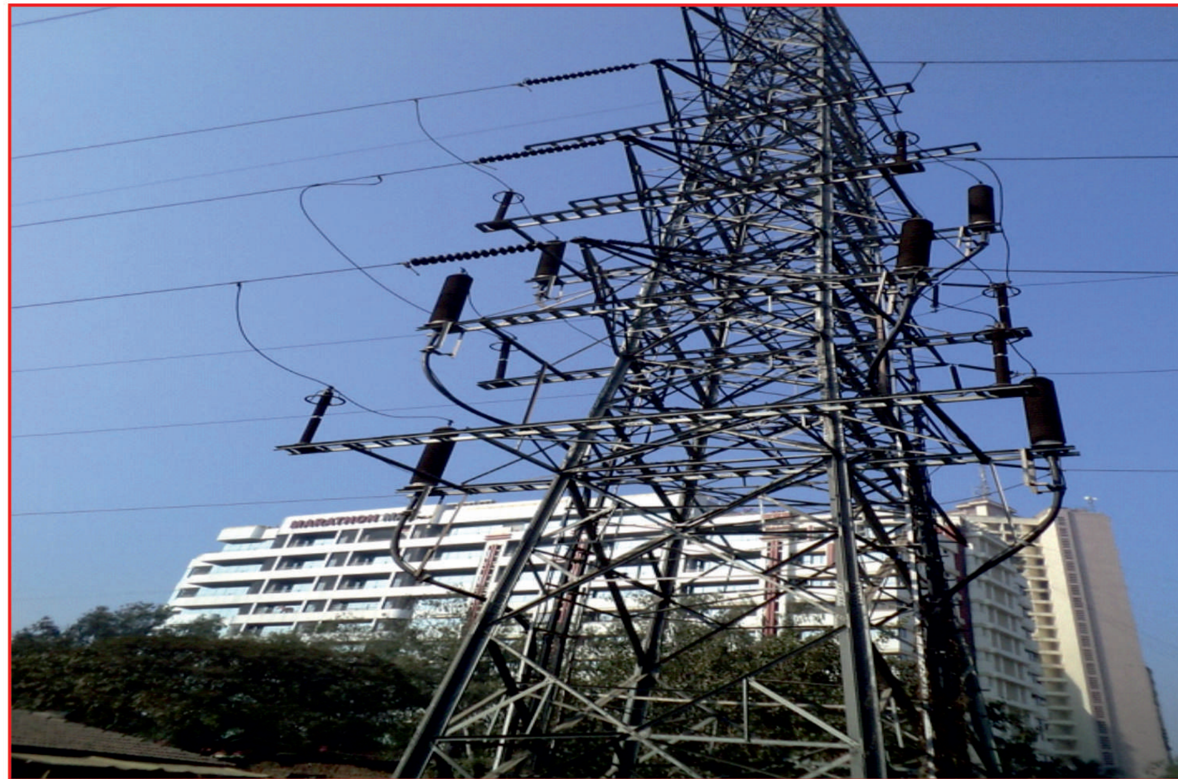
Cable Termination Tower (Multicircuit)
